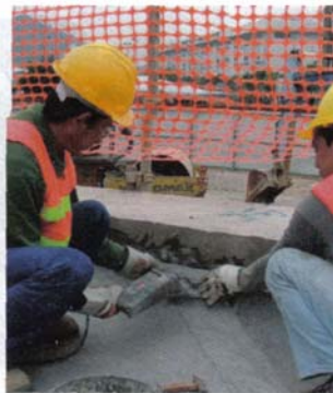
Facing page: the aviation storage facility at Chek Lap Kok Airport is one of the world's largest, supplying up to 59,000l/min to aircraft. Centre left: Granular fill is placed on the geosynthetic barrier and compacted. Left: The prehydrated bentonite membrane is fixed to the tanks' ring beams.
